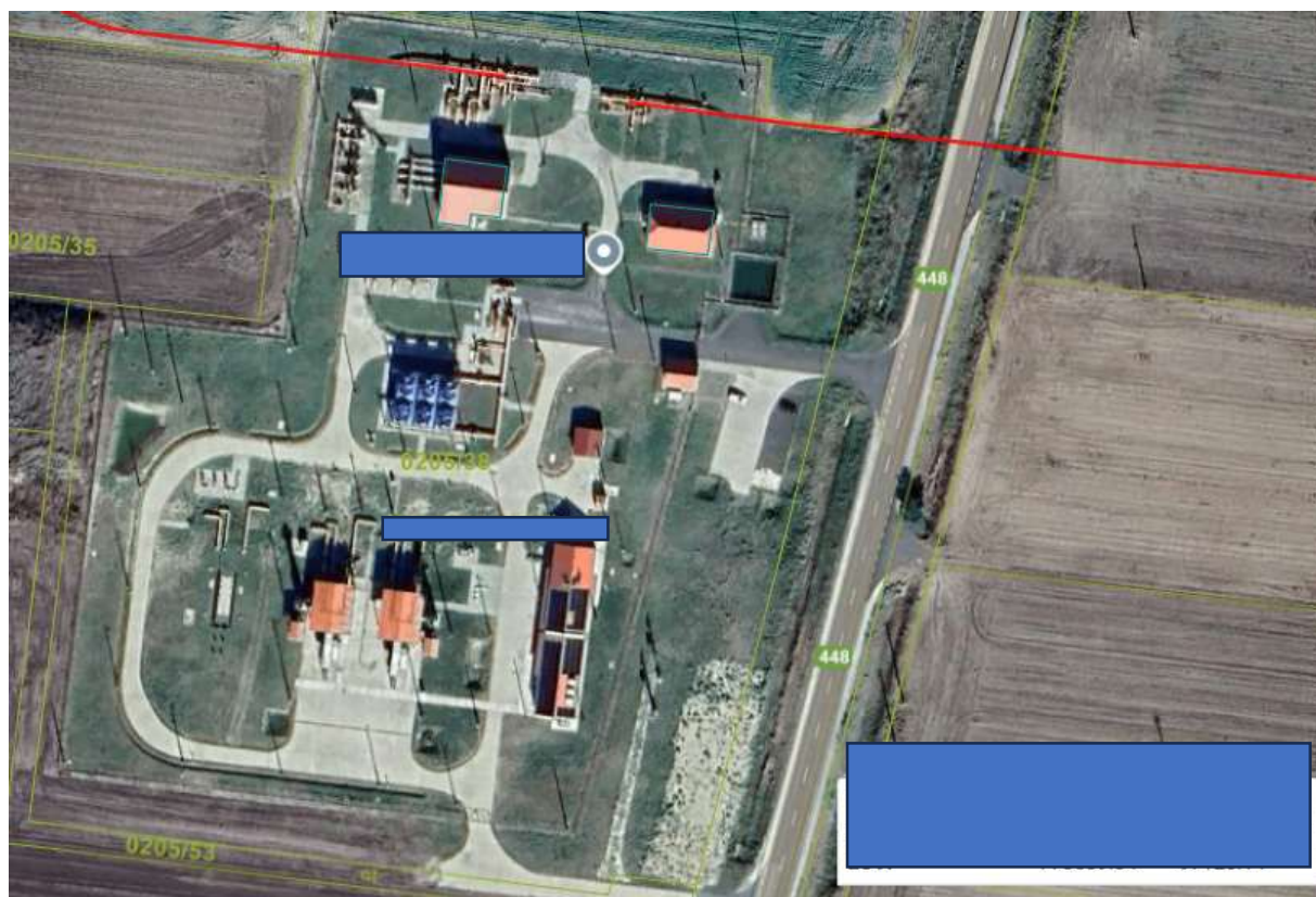
Location and coordinates of the station
