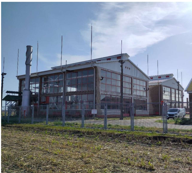
Gas turbine driven compressor units in halls at the station
